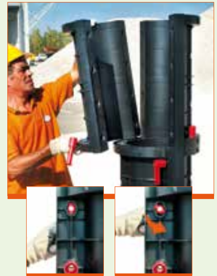
Handles lock the units into position with a 90° turn
