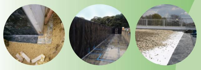
DUAL SEAL® HDPE and Sodium Bentonite laminate form a tough sheet membrane. It is easy to apply on below ground civil engineering constructions, sub level walls, cut and cover tunnels and under structural slabs and subways.
